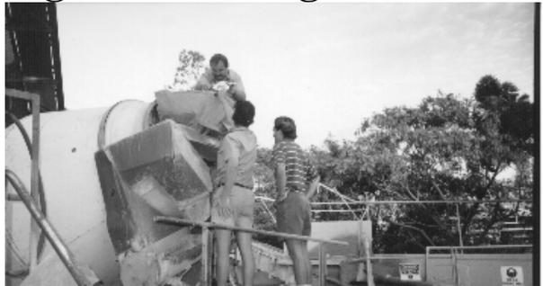
*Scanfibre steel fibres are glued into bundles, making the dosing and mixing process easy and reliable. The glue will be softened by the mixing water. Scanfibre fibres correctly dosed should never ball, even at very high dosages.*
