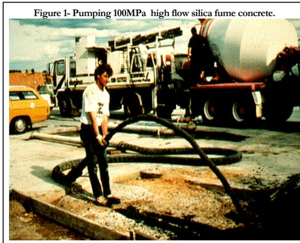
Figure 1- Pumping 100MPa high flow silica fume concrete.
