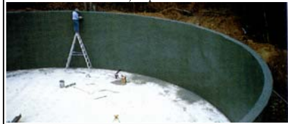
Fig 1b - Water tanks 20m diameter and 5m tall have been constructed in one day with silica fume shotcrete. An internal shutter about 3m long and full height is moved like a horizontal jump form.
