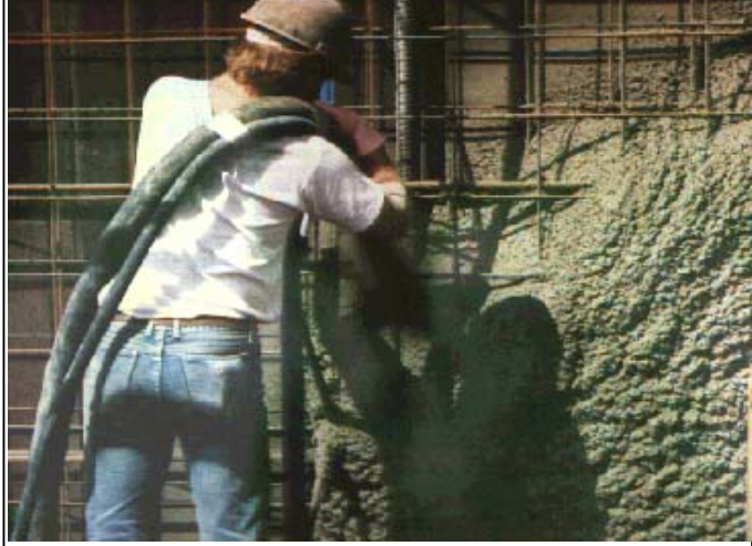
Fig 9 – Silica fume Shotcrete, the rapid simple way of applying concrete
