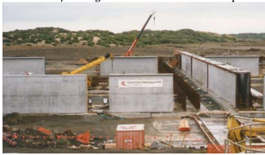
Fig 6 – Silica fume SRC was used for Blackrock sewage works. With the facility only 500 metres from Bass Strait, all concrete used was subject to high levels of chlorides as well as sulphates
